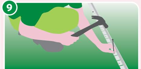
9 Once satisfied with the positioning of the Link Edge, hammer the spikes firmly into the ground.
